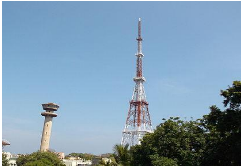
Television Tower of Doordarshan Kendra, Chennai
